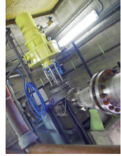
Recycle and Pressure Control Valve
