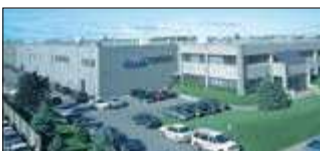
Montreal, Canada Velan Inc., Plant 2 and 7
