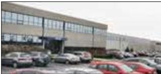
Montreal, Canada Velan Inc., Plant 1
