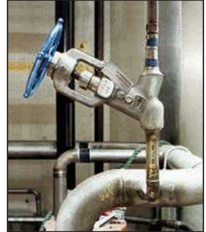
In-service photo of Class 2500 hermetically-sealed Y-pattern bellows seal valve.
